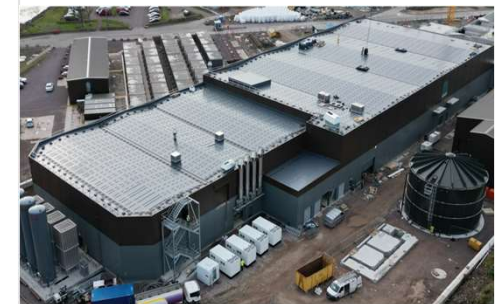
Applecross - Construction 7m smolt at 500g 29,300m 3 capacity
